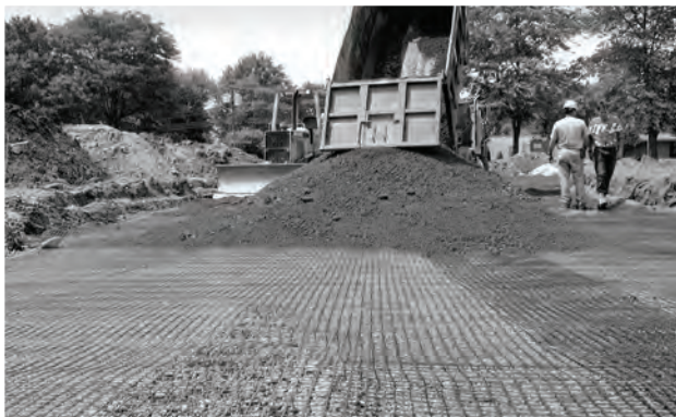
Image 9a: End dumping aggregate fill on top of Tensar Geogrid over soft subgrade.
