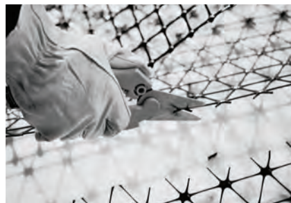
Image 6: Cutting Tensar® TriAx® Geogrid is easily achieved.
