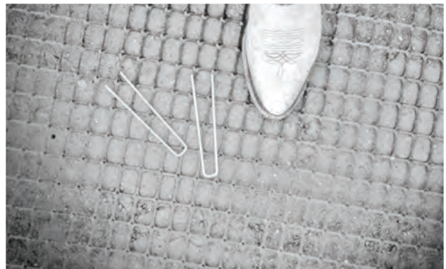
Image 7b: Staples for anchoring BX Geogrid (optional).
