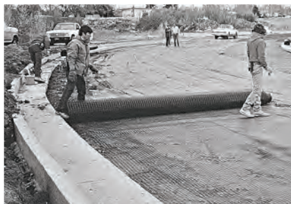
Image 5: Placing Geogrid to accommodate curves.
