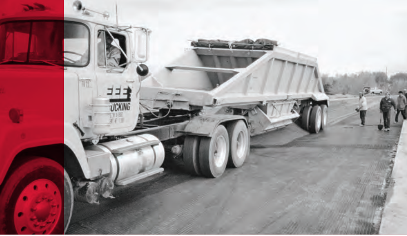
Image 8: Dumping aggregate fill on top of Tensar® Geogrid over competent subgrade.
