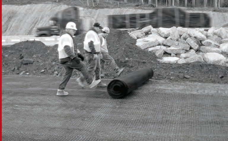
Image 3: Rolling out Tensor® Geogrid.
